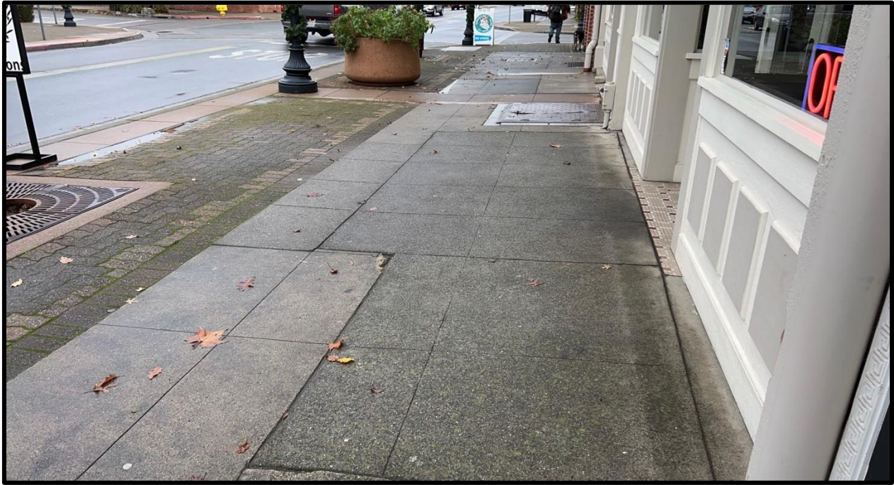
Figure 1: Existing Sidewalk on Montgomery Street
